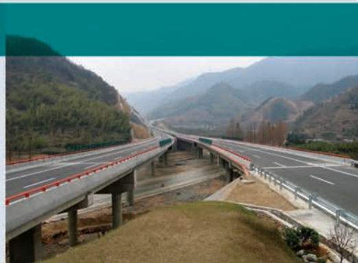
Autopista Ningbo-Shengz Zhou (China)
