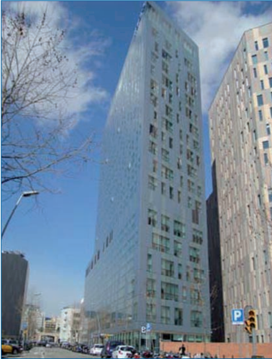
Hotel Novotel Diagonal. Barcelona
